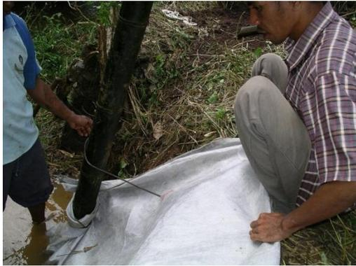
Protection by gabion stone cages can be further improved with geotextile tissue which lets water flow through but retains the soil particles. This will no doubt help to avoid soil being eroded behind the stone filled gabions.
