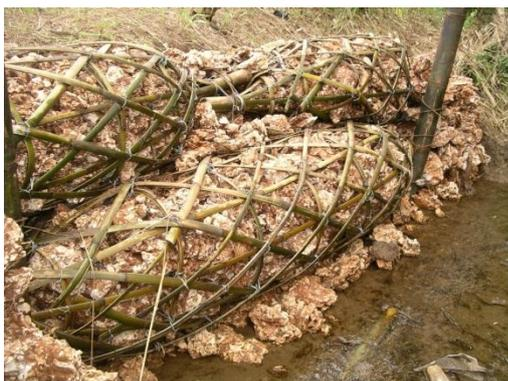
We opted for a spool-shaped gabion design which easier should resist violent storm water impact. In addition a retainer bar system anchors the gabions into the river bank. The stack of gabions leans at 80° against the river banks and creates by its weight a certain pressure to hold the soil in place.
