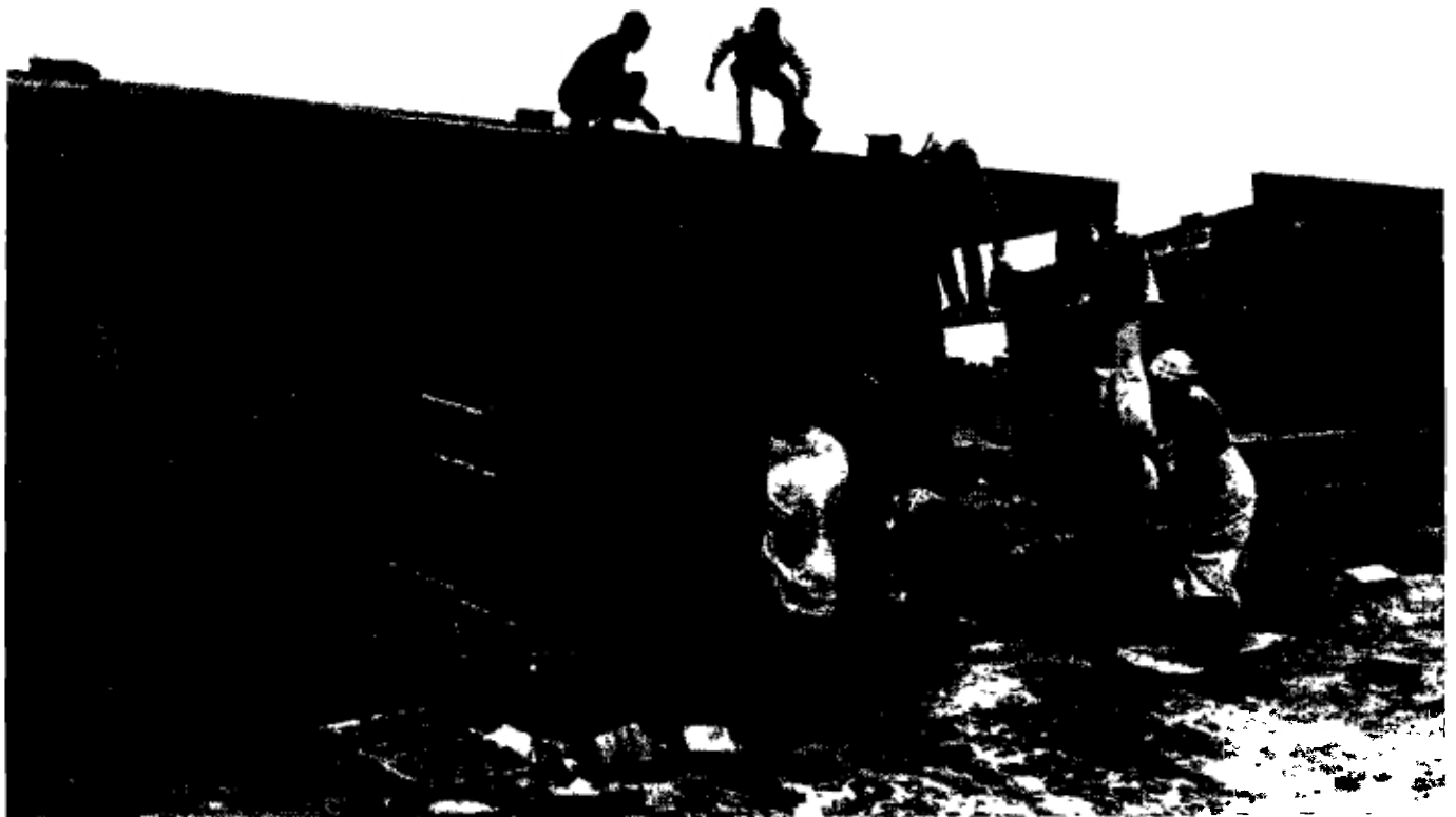
Autoconstrucao in Machava, a Maputo suburb. The self-help part is mainly assured by women, doing the unskilled work and assisting carpenters and masons from the project staff. The standard was high, and one house costed 1977 aprox. 130 000 MZM, at the time over 4000 USD. Photo: Eva Savfors
